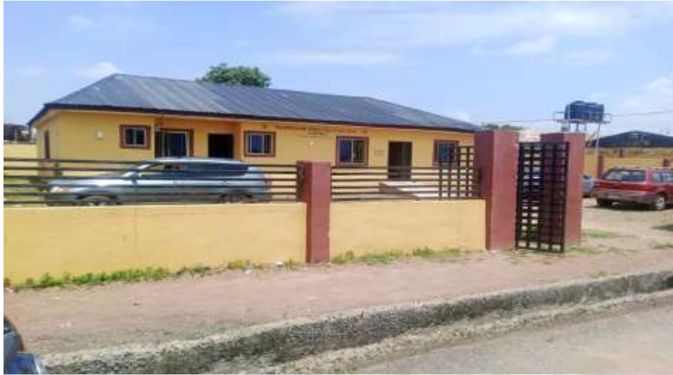
Figure 3: Upgraded Facility at Ubandawaki/ Olowo PHC Centre, Ilorin West
